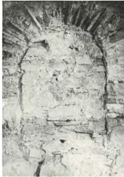
Masonry of a decorative niche of the 11th c. after removal of plaster.
