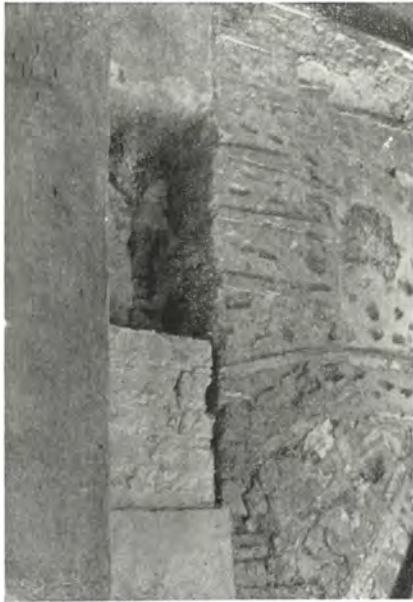
Joint between 11th and 12th cent. wall after the removal of plaster.
