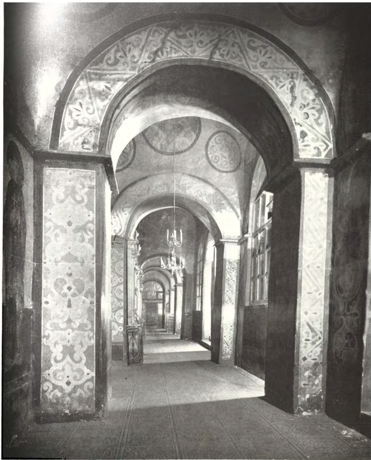
25. Western enclosed gallery (north-south).
