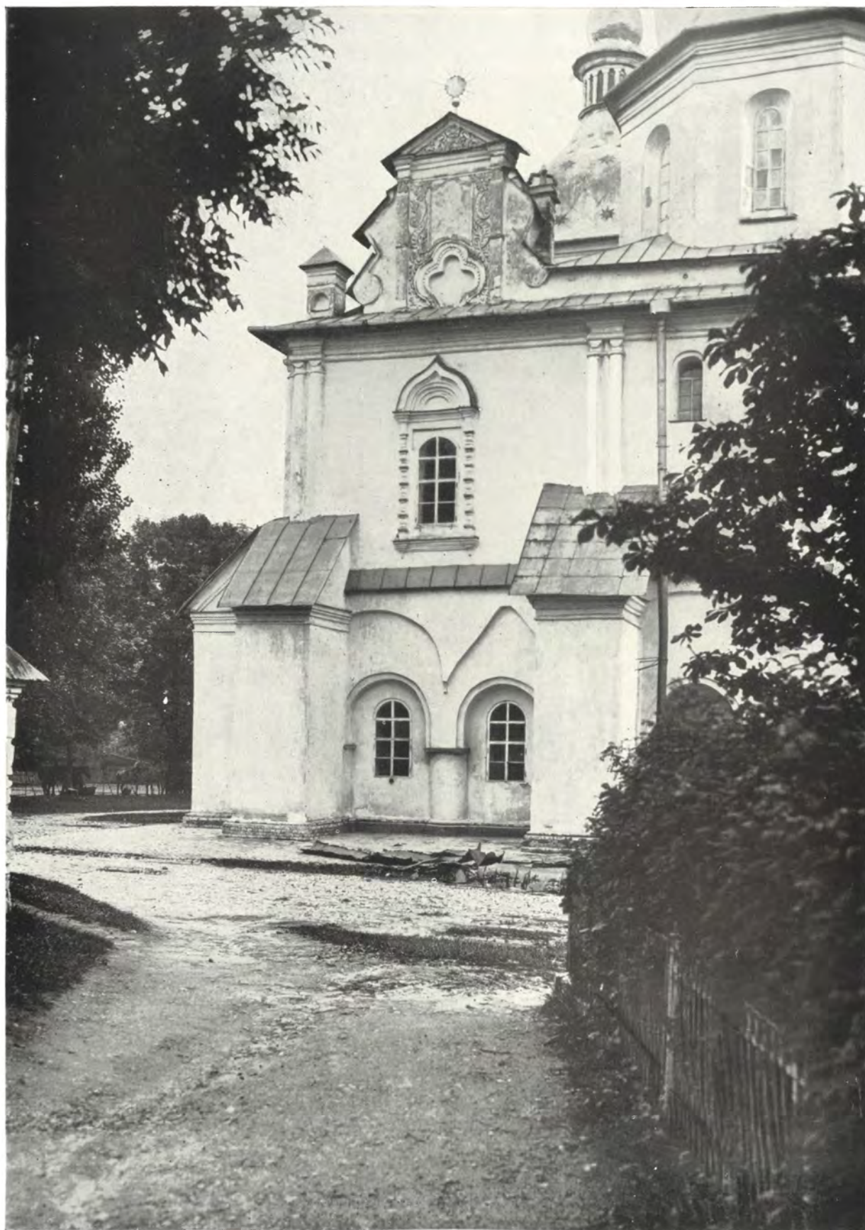
11. Part of the western façade.
