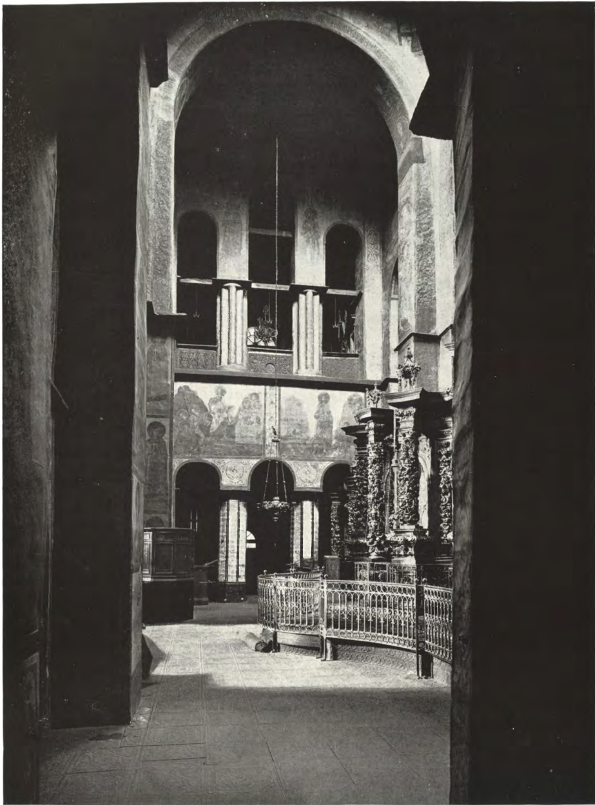
28. Interior of the Cathedral. Main transept.
